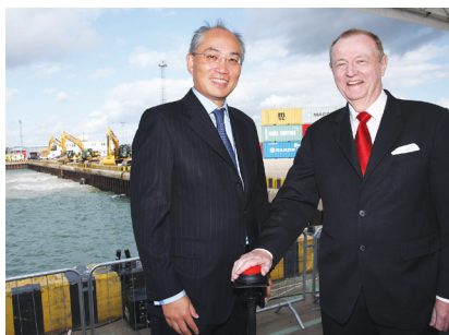
John Meredith, Group Managing Director, Hutchison Port Holdings (HPH), (right), accompanied by Clemence Cheng, Managing Director, HPH Central Europe, initiates work to reclaim The Port of Felixstowe's Dock Basin to construct the new Felixstowe South container Terminal.
